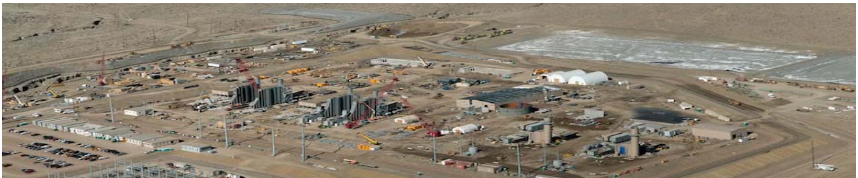
Construction progress at Pueblo Airport Generation Station as of 3/31/11
